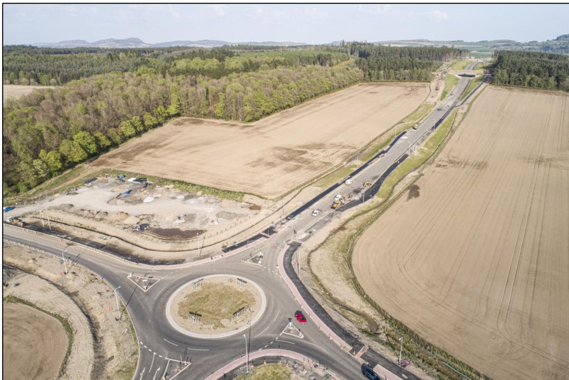
A94 Roundabout and New Kingsway Progress May 2024
