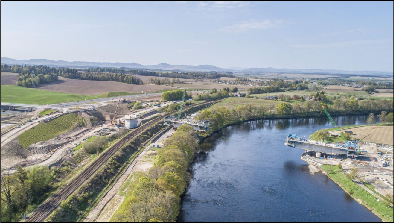
Destiny Bridge Progress May 2024
